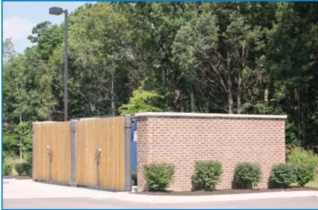
A combination of building materials and landscaping effectively screen a dumpster pad.
