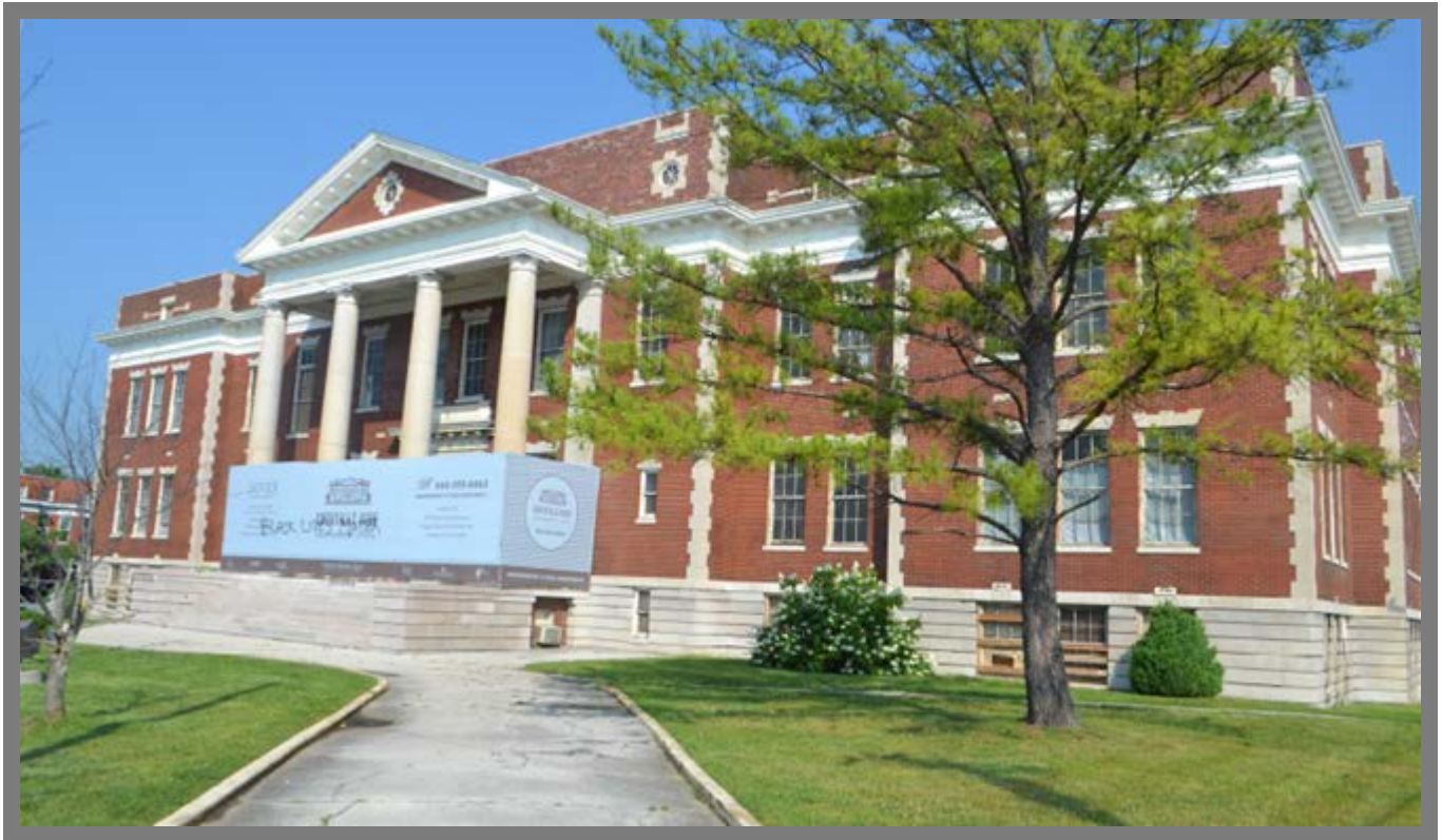
Historic Knoxville High School 2016 – pre-renovation
