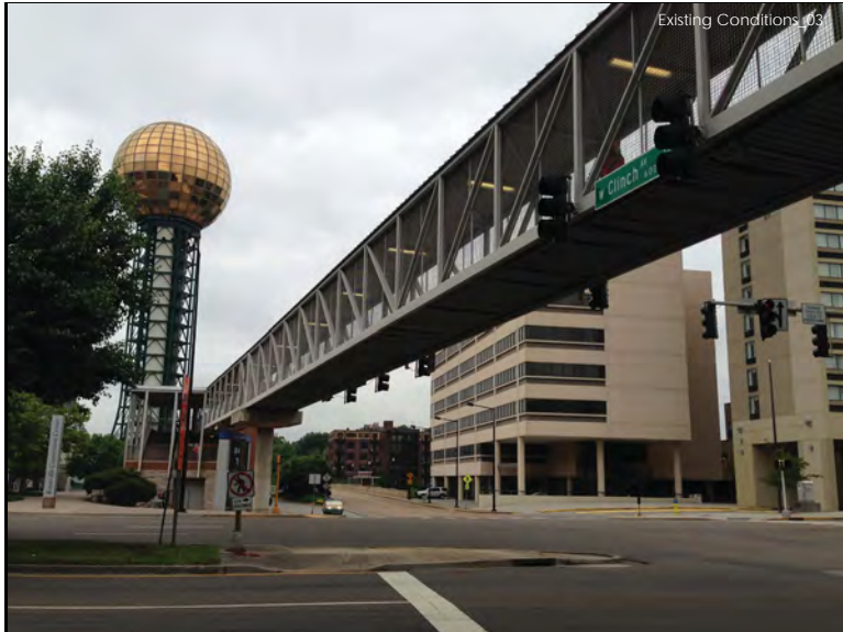
Existing view from Henley Street, looking west
