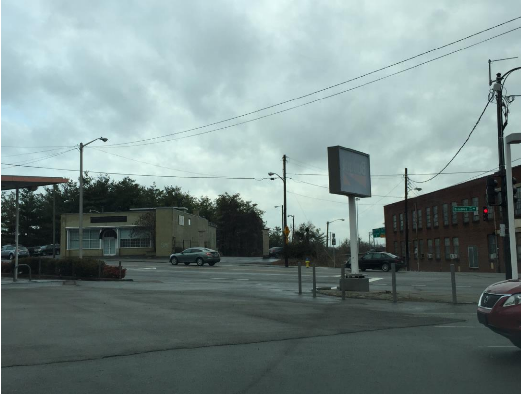
1 Existing pole sign to be refurbished and new sign faces installed.
