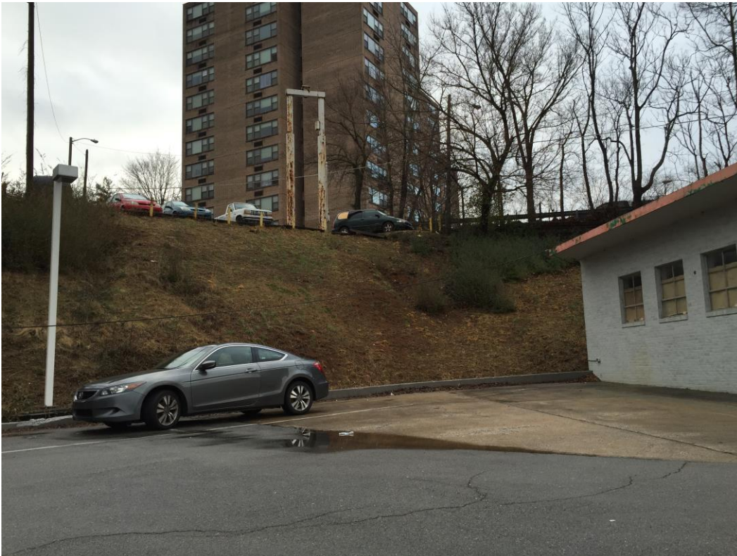
2 Sign structure at top of hill to be refurbished and new sign attached.
