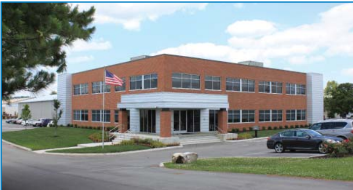
The Technology for Energy Corporation underwent an expansion and facade renovation in 2012.
