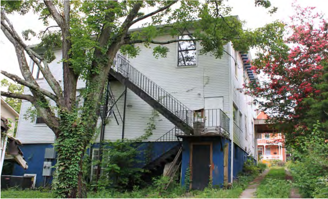
Picture 2 - 930 Luttrell – Rear elevation
