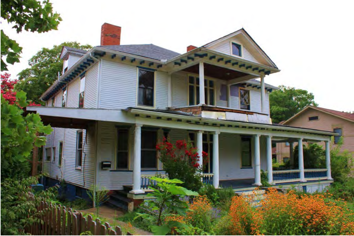
930 Luttrell – Front, northwest view
