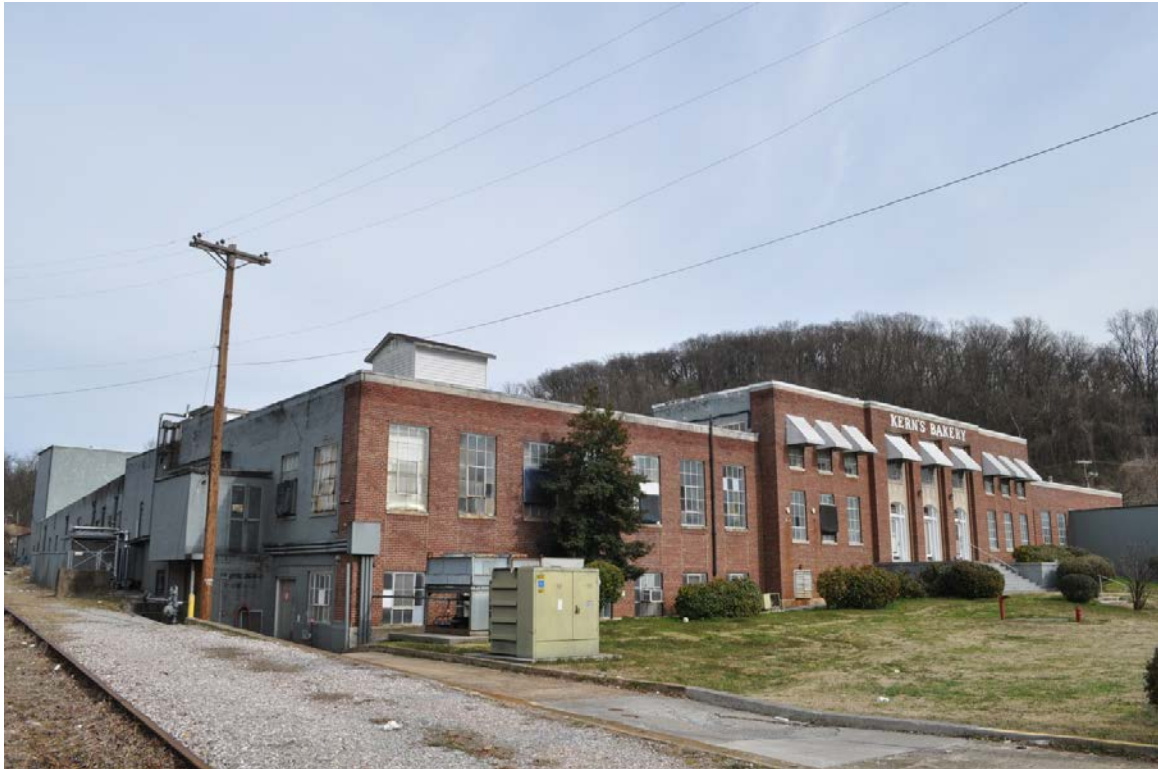
Kerns Bakery – North facade
