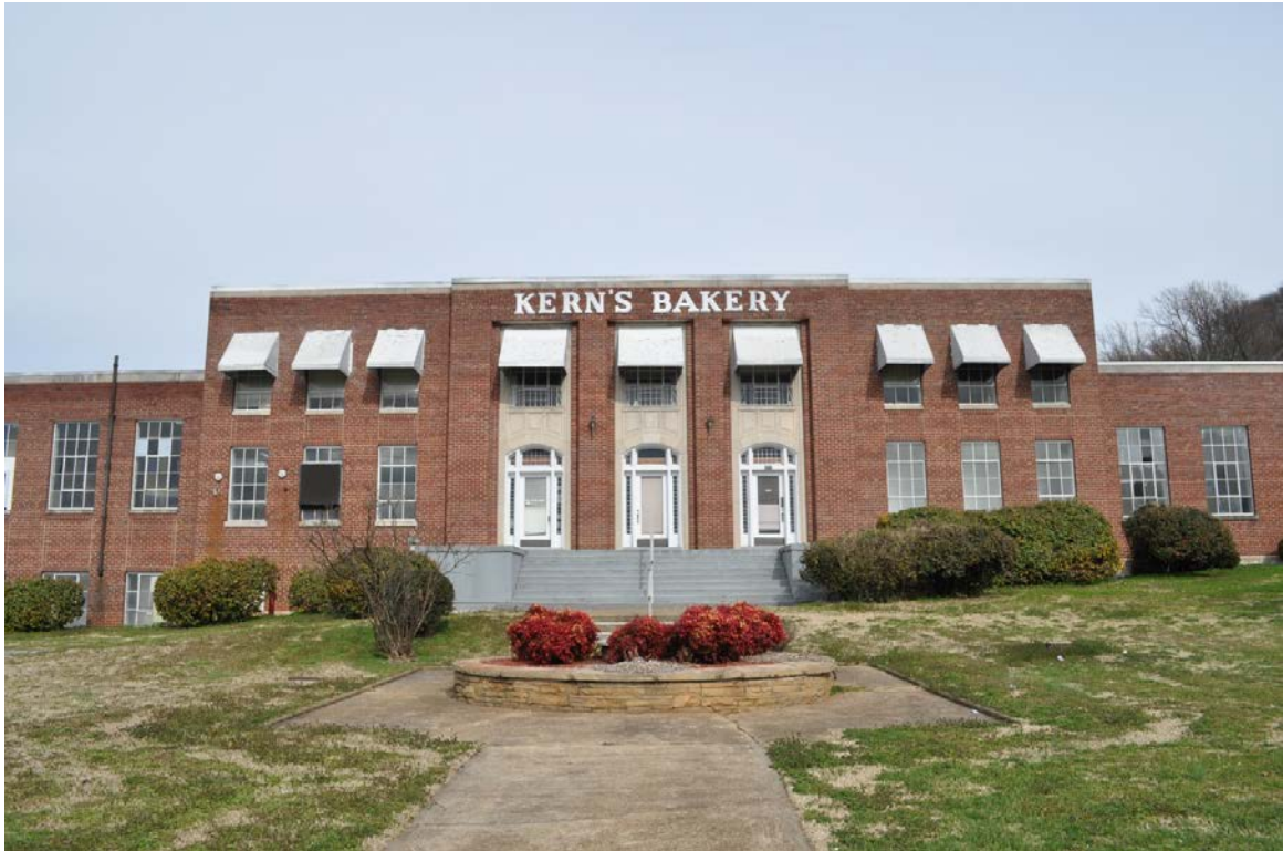
Kerns Bakery – Front façade, center section
