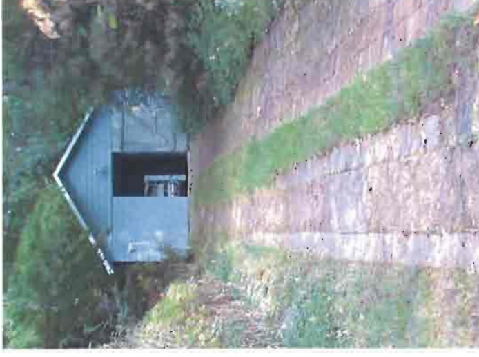
This split driveway with a grass median reduces the amount of impervious pavement surface.
