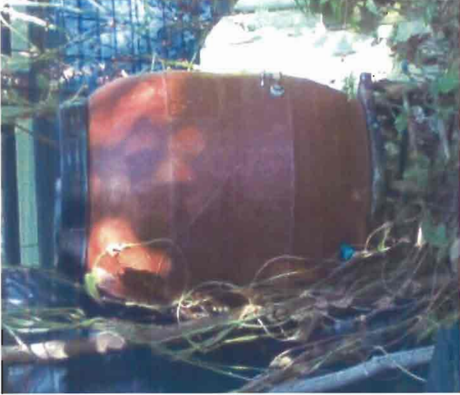
Rain barrel used to capture storm water for irrigation purposes.
