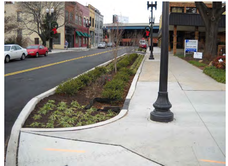
Streetscape improvements to North Gay Street included new sidewalks, lighting, on-street parking, and bio-retention that infiltrate stormwater and includes landscaping.
