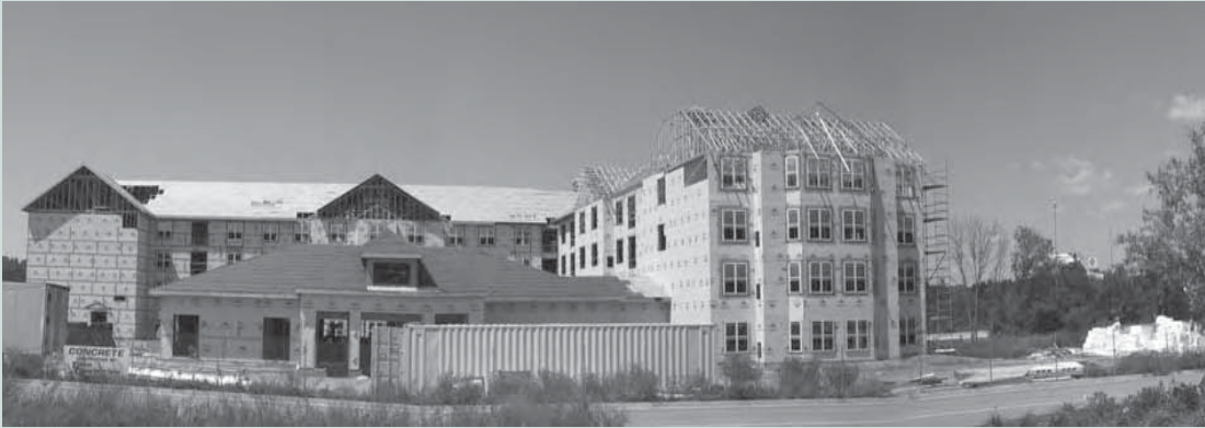
Construction continues at the Turkey Creek mixed-use development.
