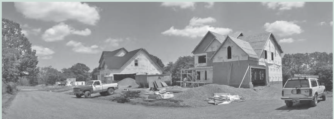
Construction in the Southwest County Sector at the Turnberry Subdivision
